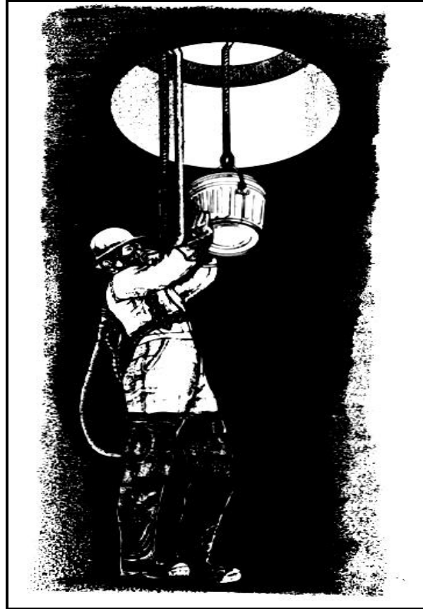
Figure 12-23. Removing sludge
