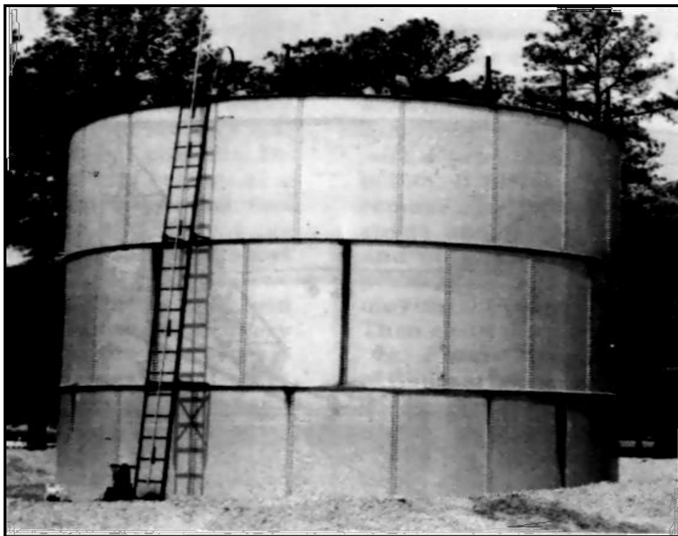
Figure 12-2. Bolted steel tank
