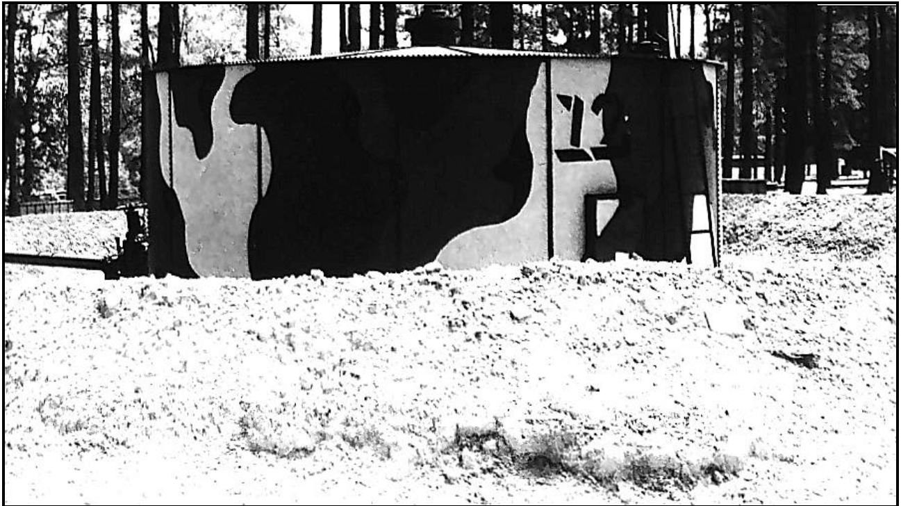
Figure 10-1. Earthen firewall
